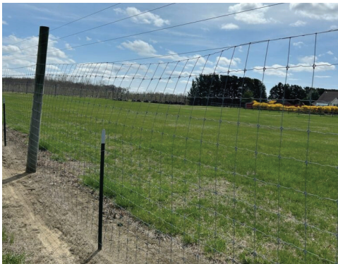
Figure 4. The deer jumped through the 8-foot catch wire. A 2-foot straight wire fence above 6 feet of woven-wire fencing was ineffective. Photo by H. Gohil
