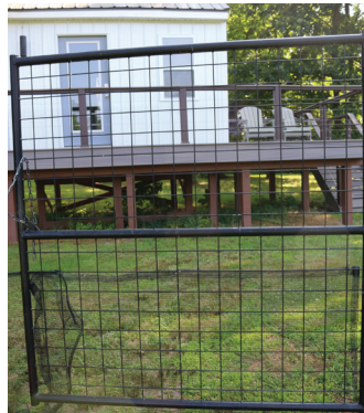
Figure 5. Netting to cover the space under the gate. Photo by H. Gohil
