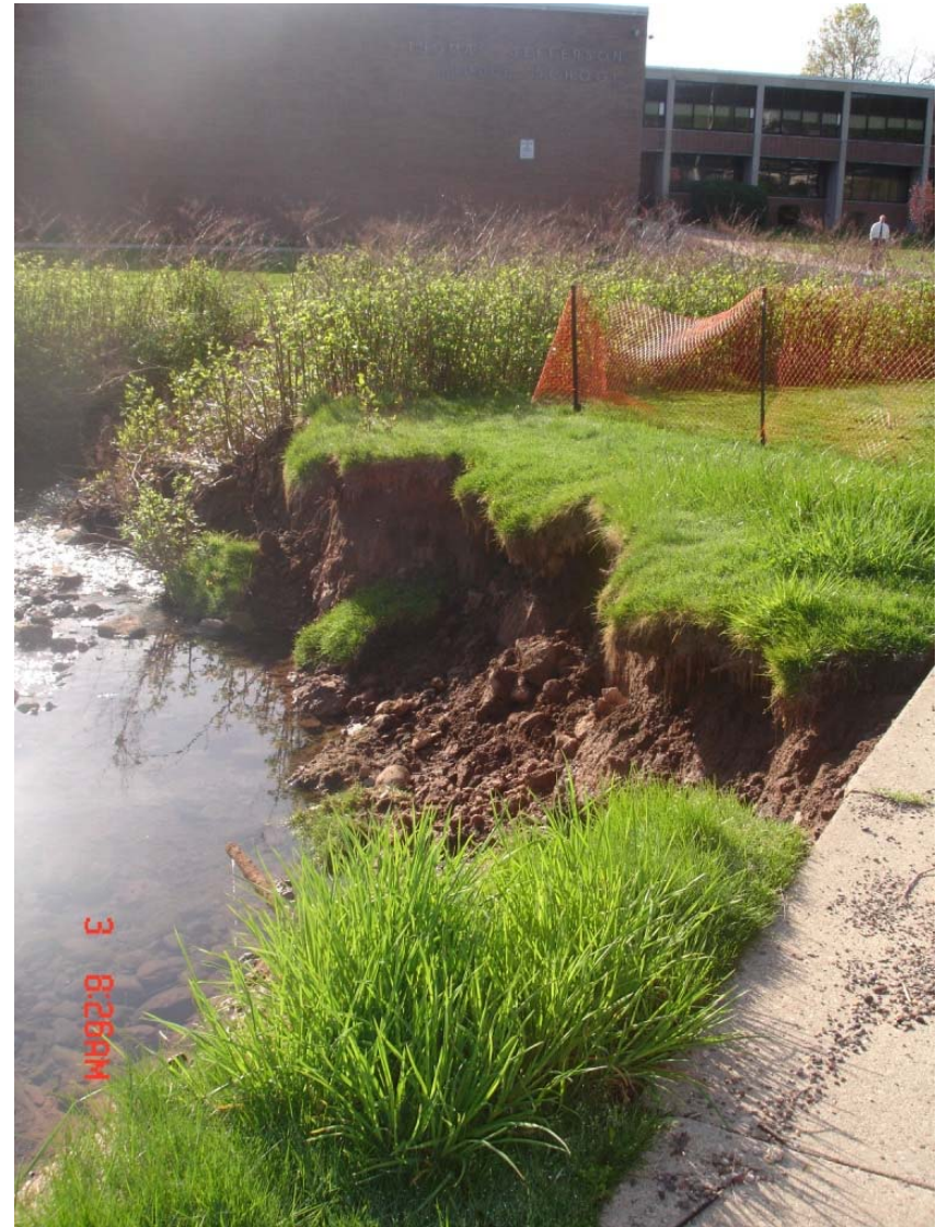
Figure 4. Erosion downstream of discharge pipe at Thomas Jefferson Middle School.
