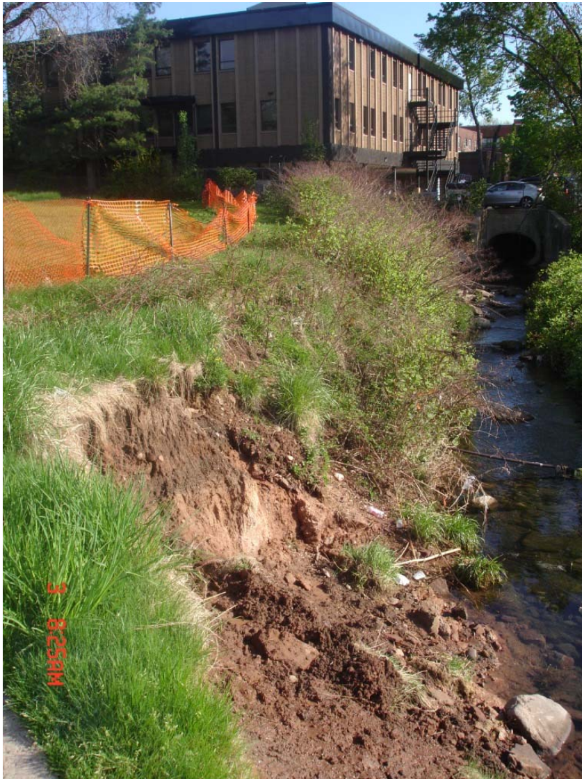
Figure 4. Erosion downstream of discharge pipe at Thomas Jefferson Middle School.
