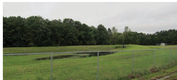
Figure 8. A retention basin collects water shed from the GE landfill and the eastern portion of the Voorhees landfill.
