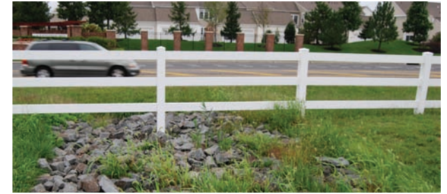
Figure 13. A stone-bottom swale directs water into a deeper swale which channels water toward the pond.
