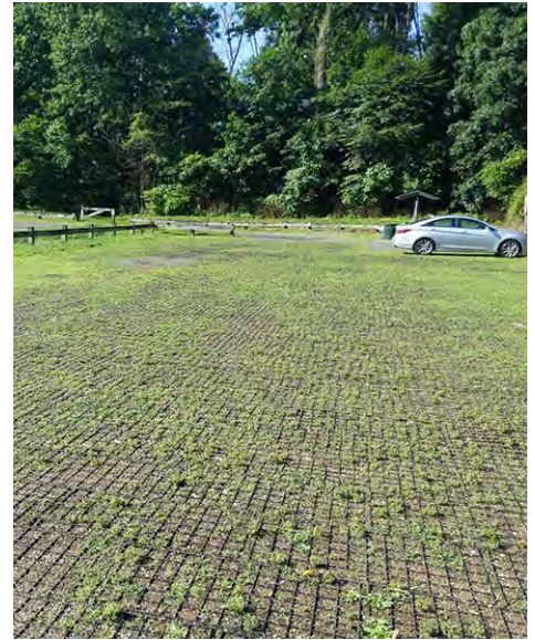
Figure 4.20: Pervious Parking.
