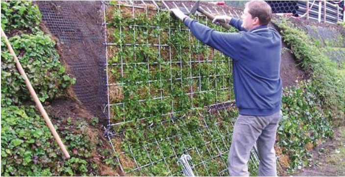
Figure 3.4.8 Erosion Mat
