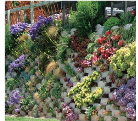
Figure 3.4.13 Plantable retaining wall
