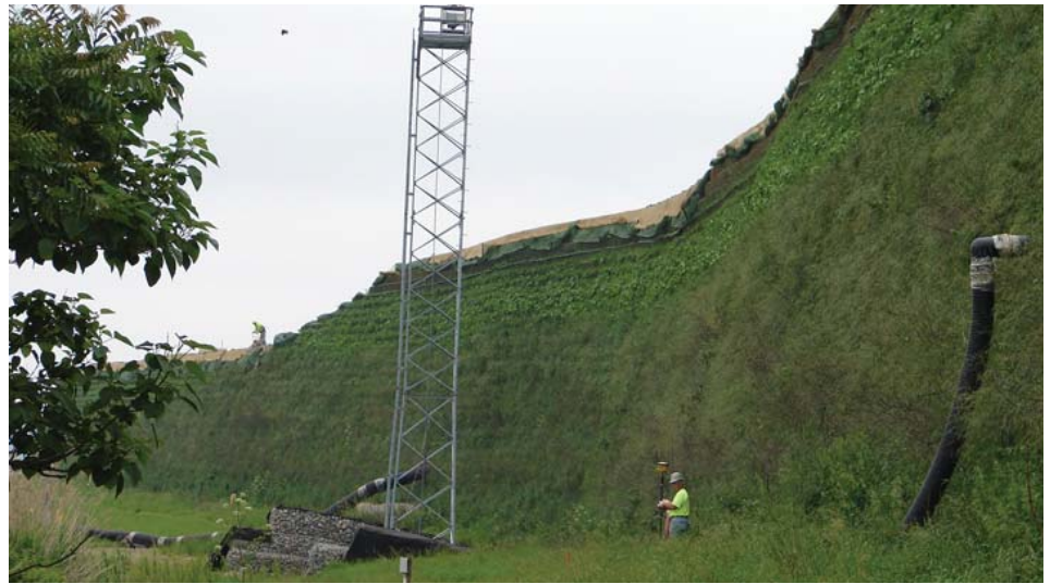
Figure 3.2.4. Example of a MSE berm at Cherry Island Landfill.
