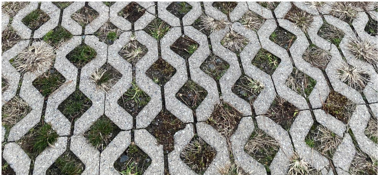
Figure 3.38: Permeable Walking Path at John A. Phillips Open Space Preserve, Old Bridge
