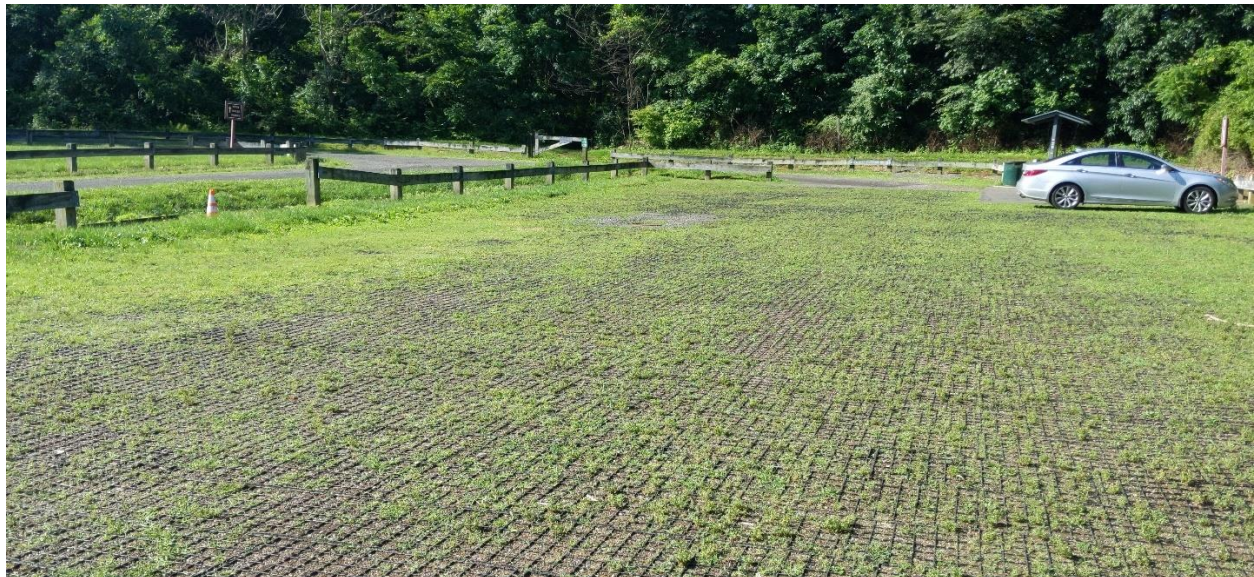
Figure 3.37: Permeable Parking Installation in Mercer County Parks at Baldpate Mountain.
