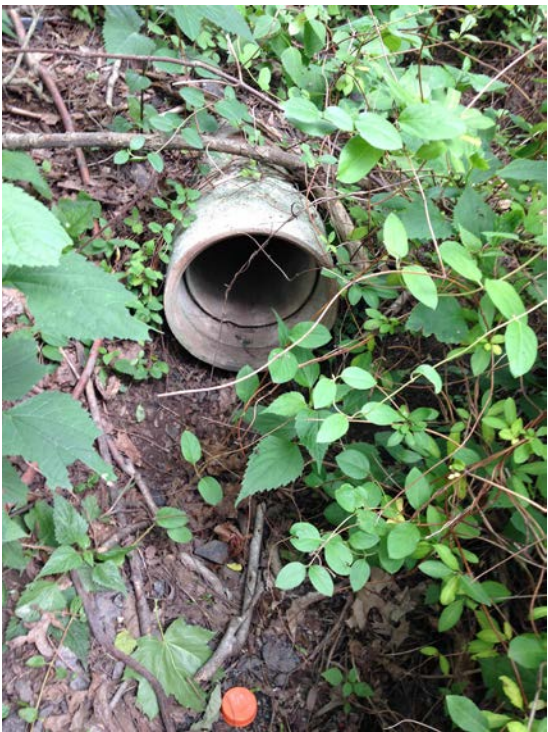
Typical Discharge Pipe.
