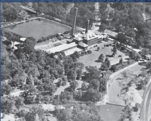
The intake basin on the west side of Van Buskirk Island may seem like a natural leg the in the Hackensack River, but it is a manmade extension first built to service the J & H Van Buskirk grist mill. In this image you can see the intake basin being modified to be the temporary coagulation basin before the 1905 coagulation basin, located top left, under went extensive renovations.
