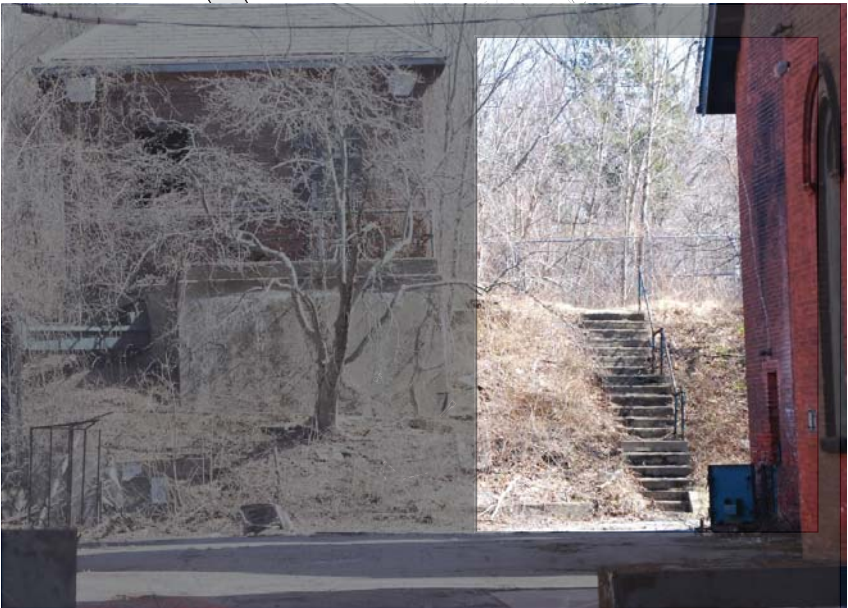
Gate House stairs: 20 risers and 2 landings
