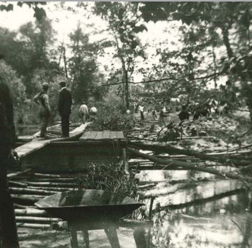
In 1901 the Water Company purchased Veldran’s Mill, located about a half of a mile north of Van Buskirk Island. A dam was built with a water storage capacity of 1.4 billion gallons of water, enough to supply 35 million gallons daily to the Water Works. This constant supply was now available with no fluctuation due to rainfall or seasonality in water flows. The picture at left shows the beginning of construction in the early 20th century.
