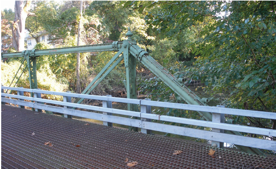
Figure 63: Elmstreet Bridge (c. 1892), Phoenix column truss
