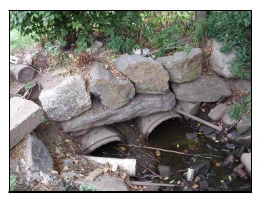
5. Elliptical culvert clogged with debris at the rear of 545 Dell Road (10/06/05)
