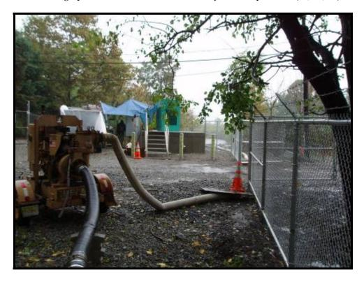
2. View of bypass pump system and new DePeyster Pump Station (10/11/05)
