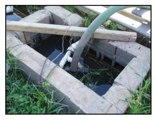
2. Sump pit for make-shift pump system at 996 Belleville Turnpike (10/06/05)
