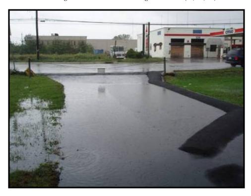
2. Looking at the raised berm and ponding of the driveway located at the south end of property (10/12/05)
