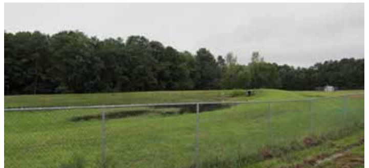
Figure 11. A retention basin collects water shed from the GE landfill and the eastern portion of the Voorhees landfill.
