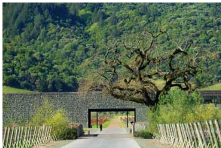
Figure 80. Dominus Winery, Yountville, California designed by Herzog and de Meuron uses gabions filled with local basalt rock.
