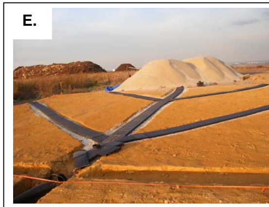
Fig. 16 A-F. Construction of USGA-type golf course field plots atop the 1 E Landfill: a. Clearing and leveling the site; b. constructing individual field plot barriers; c. assembling sand and drainage materials; d. placement of soil and sand underlying layers; e. placement and construction of drainage system; f. subgrade soil compaction.
