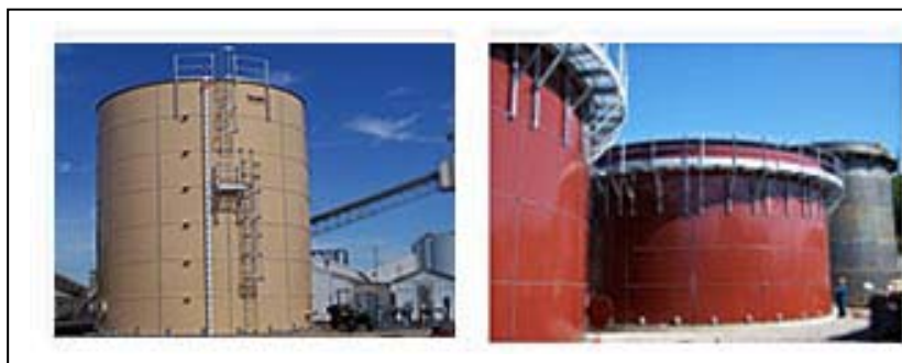
Fig. 32. Examples of above ground wastewater tanks as shown on the Liquidtanks.com web site. This company provides tanks for leachate storage.
