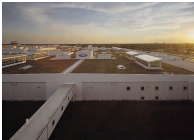
At more than 10 acres, the largest green roof in the world sits atop Ford's Rouge River Manufacturing Complex. The green roof is one component of a renovation designed to make the facility more environmentally sustainable. PHOTOS COURTESY OF GREEN ROOFS FOR HEALTHY CITIES
