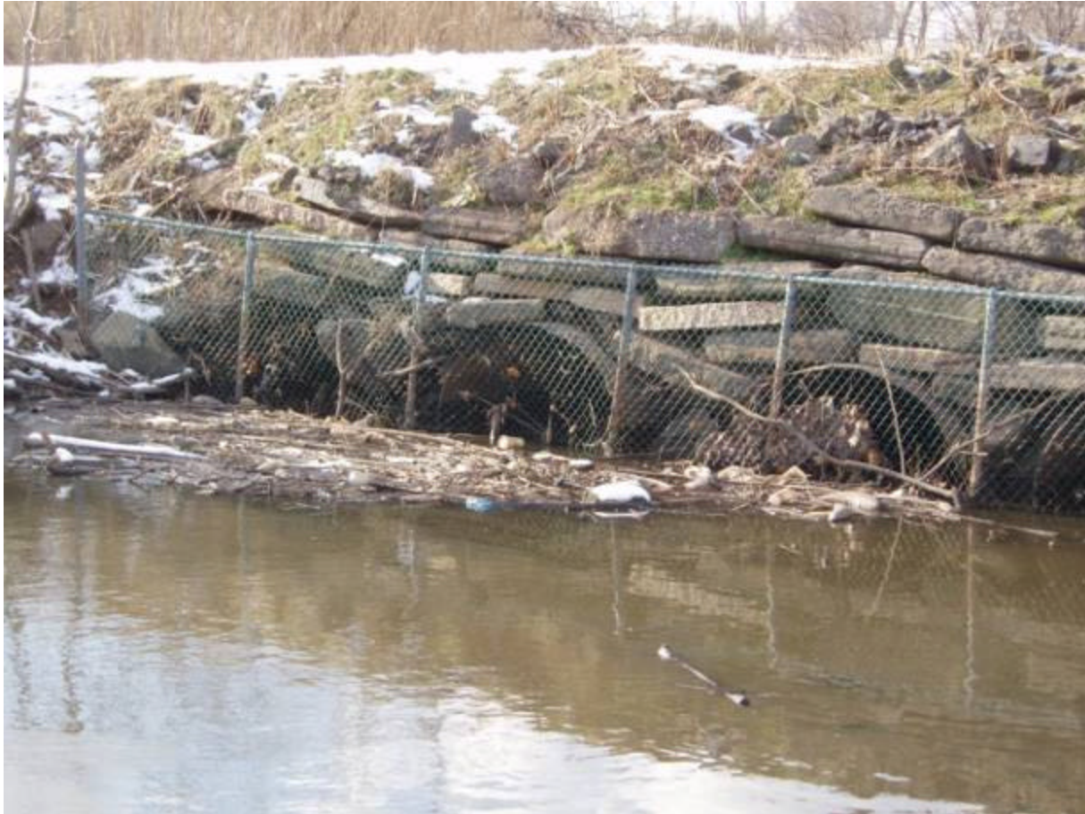
Photo 1 Description: Trash rack on upstream side of the tide gates
