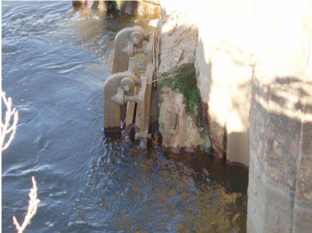
Photo 1 Description: Metal flap gate shown closed
