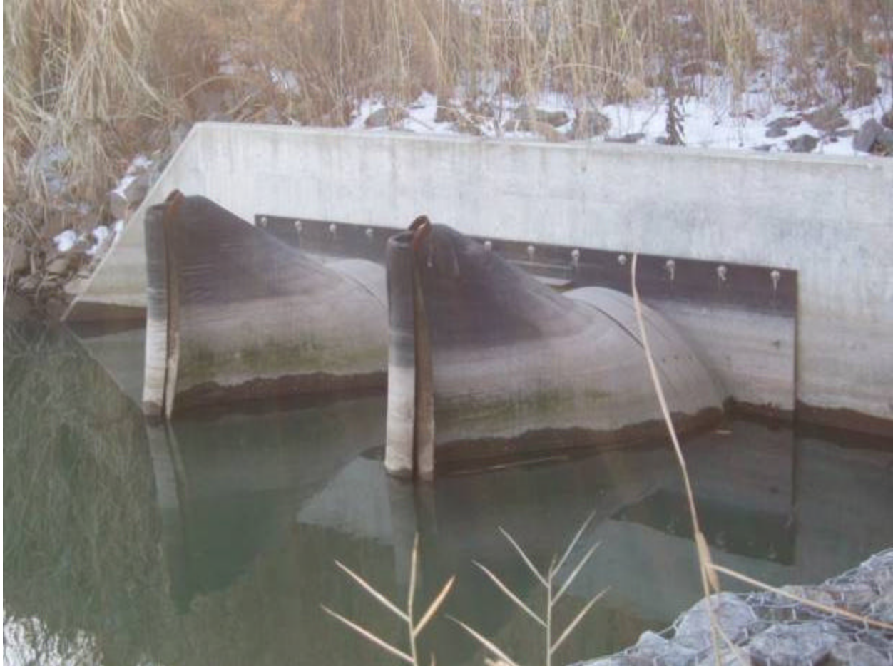
Photo 1 Description: Tideflex™ check valve structure
