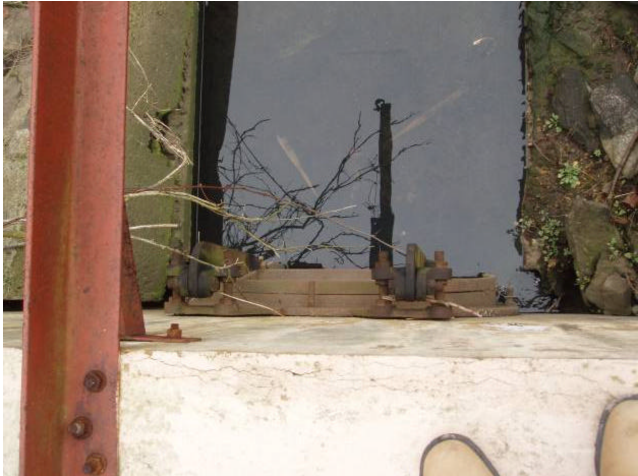
Photo 3 Description: Second 48-inch metal flap gate
