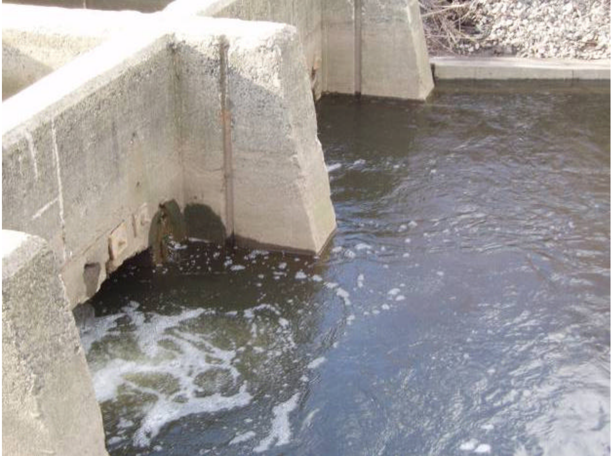
Photo 1 Description: Notice water (bubbles) traveling upstream of the tide gate during high tide conditions
