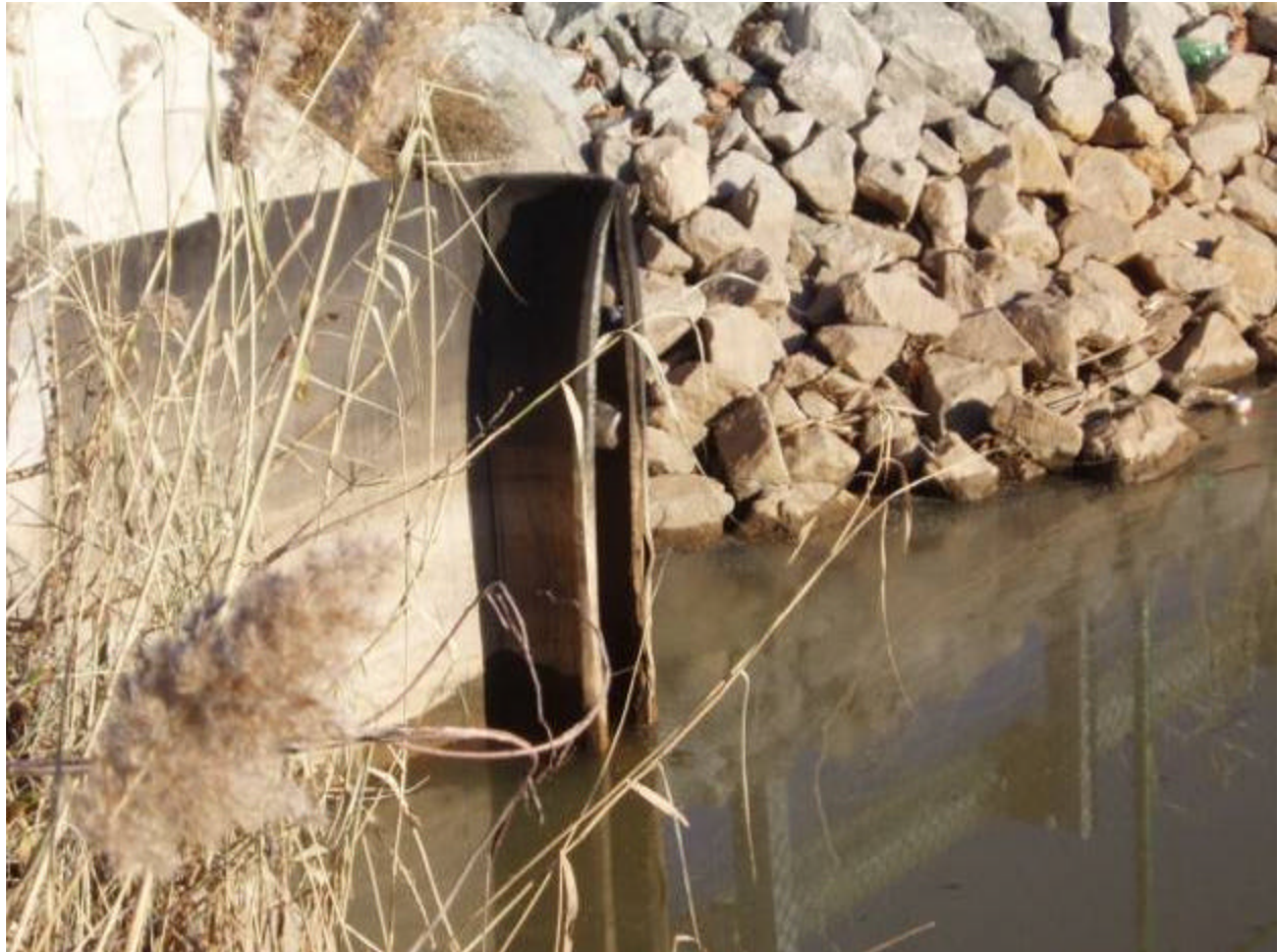
Photo 1 Description: Tideflex TM check valve structure
