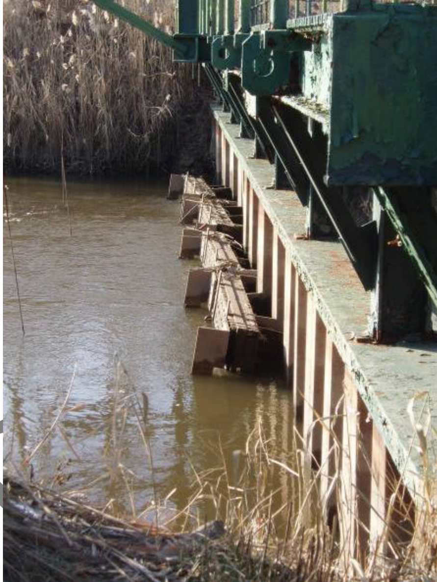
Photo 1 Description: 4 timber tide gates
