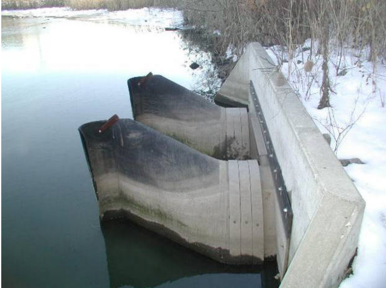
Photo 1 Description: Tideflex TM check valve structure
