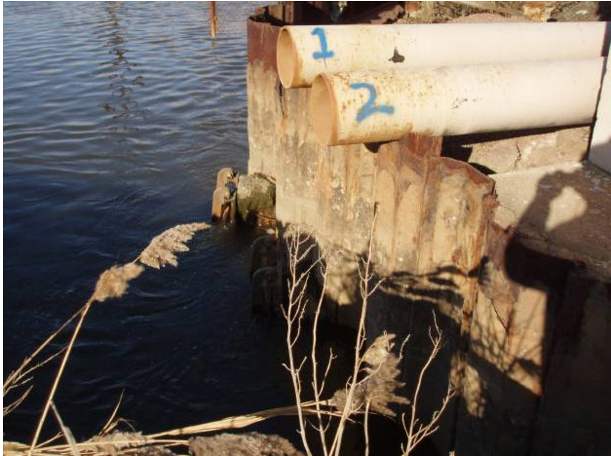
Photo 2 Description: Pump discharge pipes
