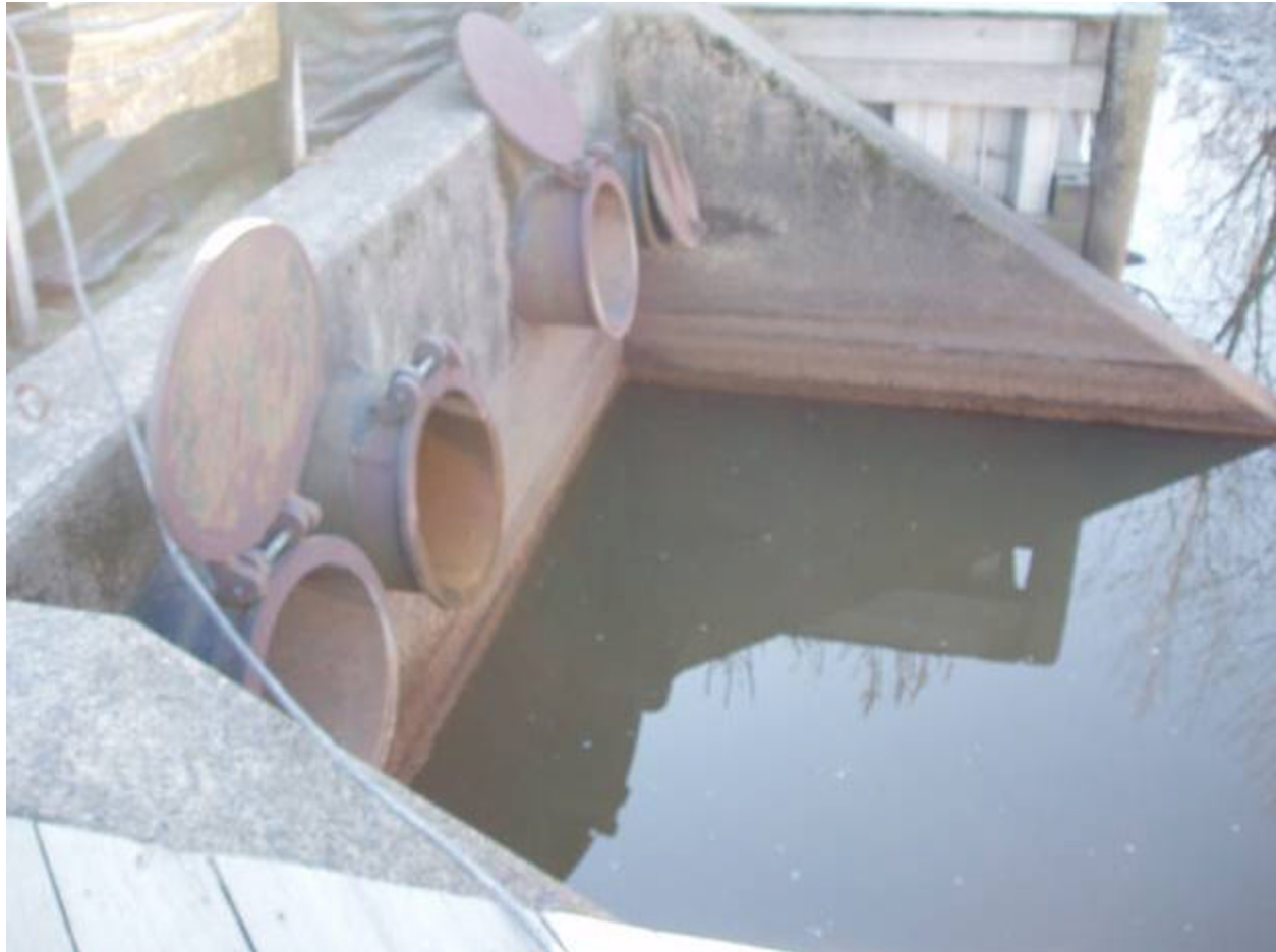
Photo 1 Description: Flap gates shown on outlet structure
