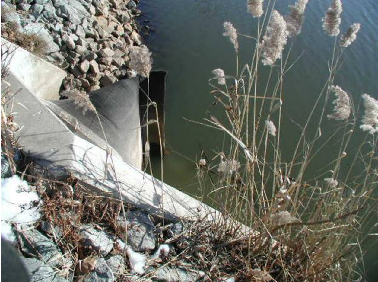
Photo 1 Description: Tideflex TM check valve structure
