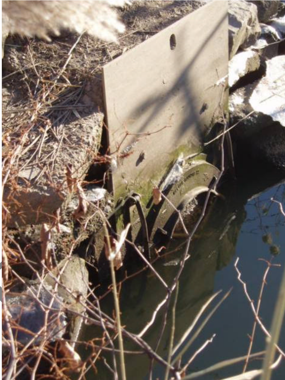
Photo 1 Description: Metal flap gate
