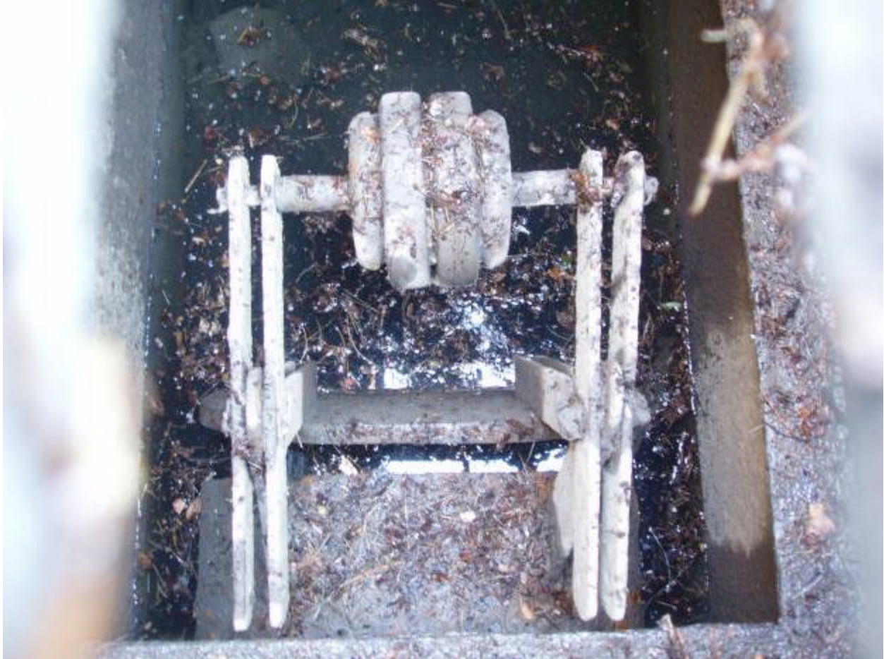
Photo 2 Description: View of metal flap gate
