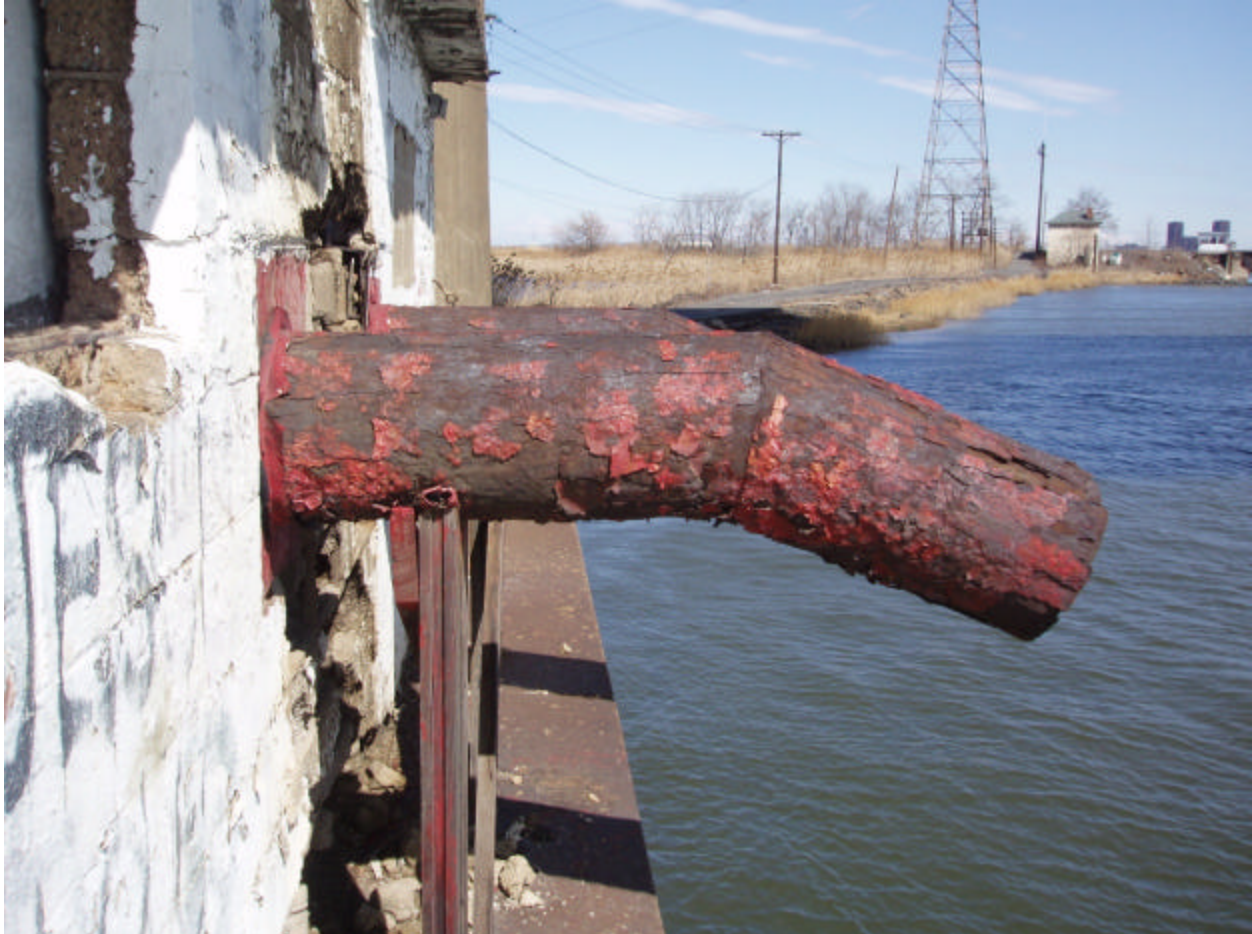
Photo 3 Description: View of discharge pipes from pump station to Hackensack River
