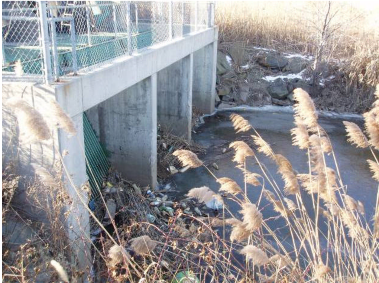
Photo 1 Description: View of trash racks at in-take structure
