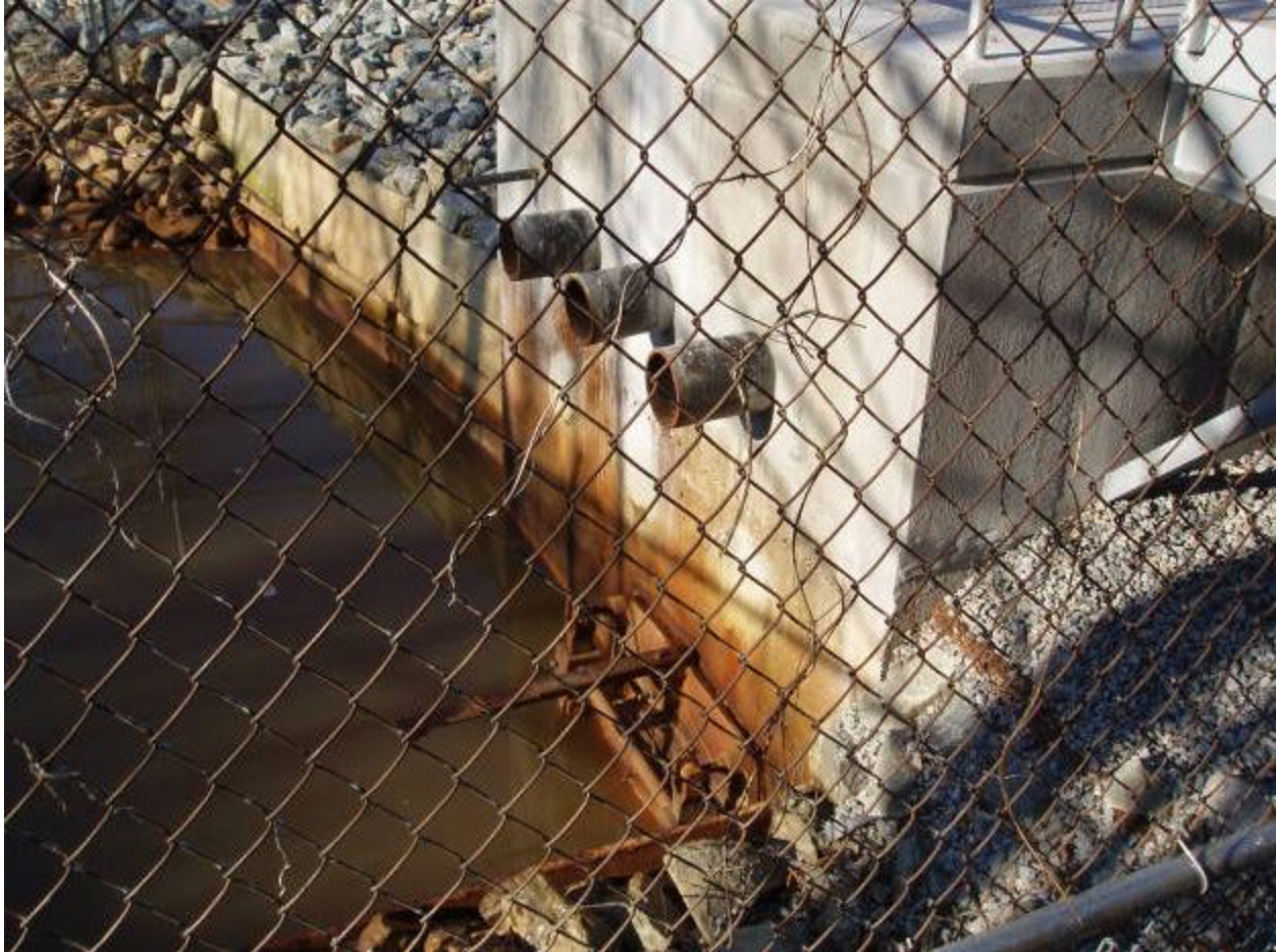
Photo 1 Description: View of tide gate and the outlet pipes for the pump station
