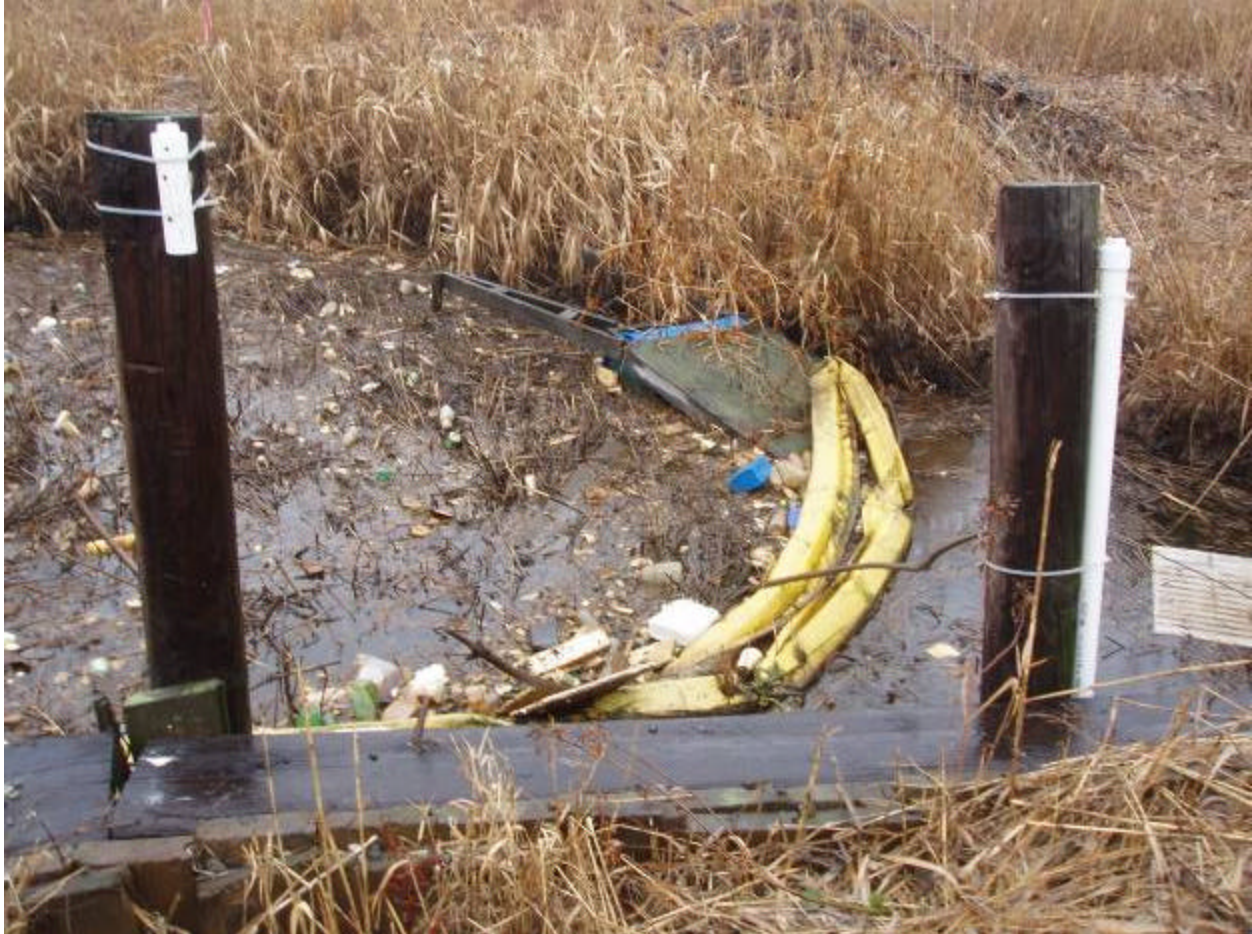
Photo 2 Description: View of trash rack on upstream side of the tide gate
