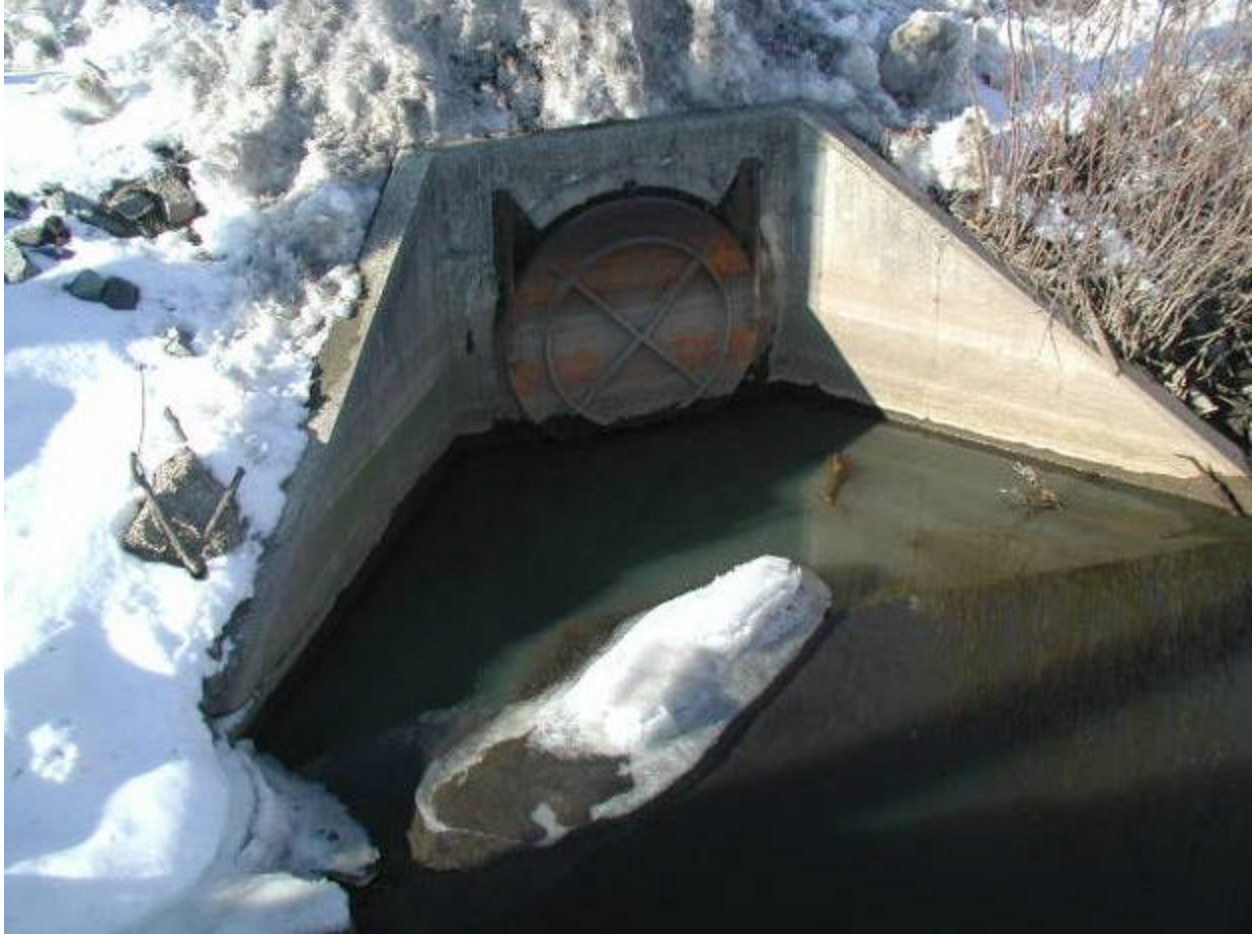
Photo 1 Description: Metal flap gate
