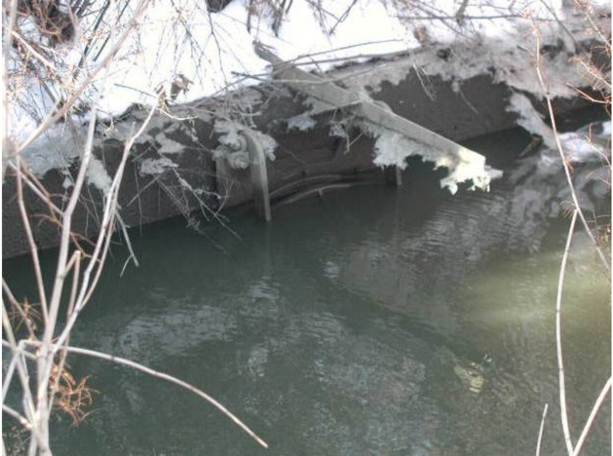
Photo 1 Description: 1 metal flap gate
