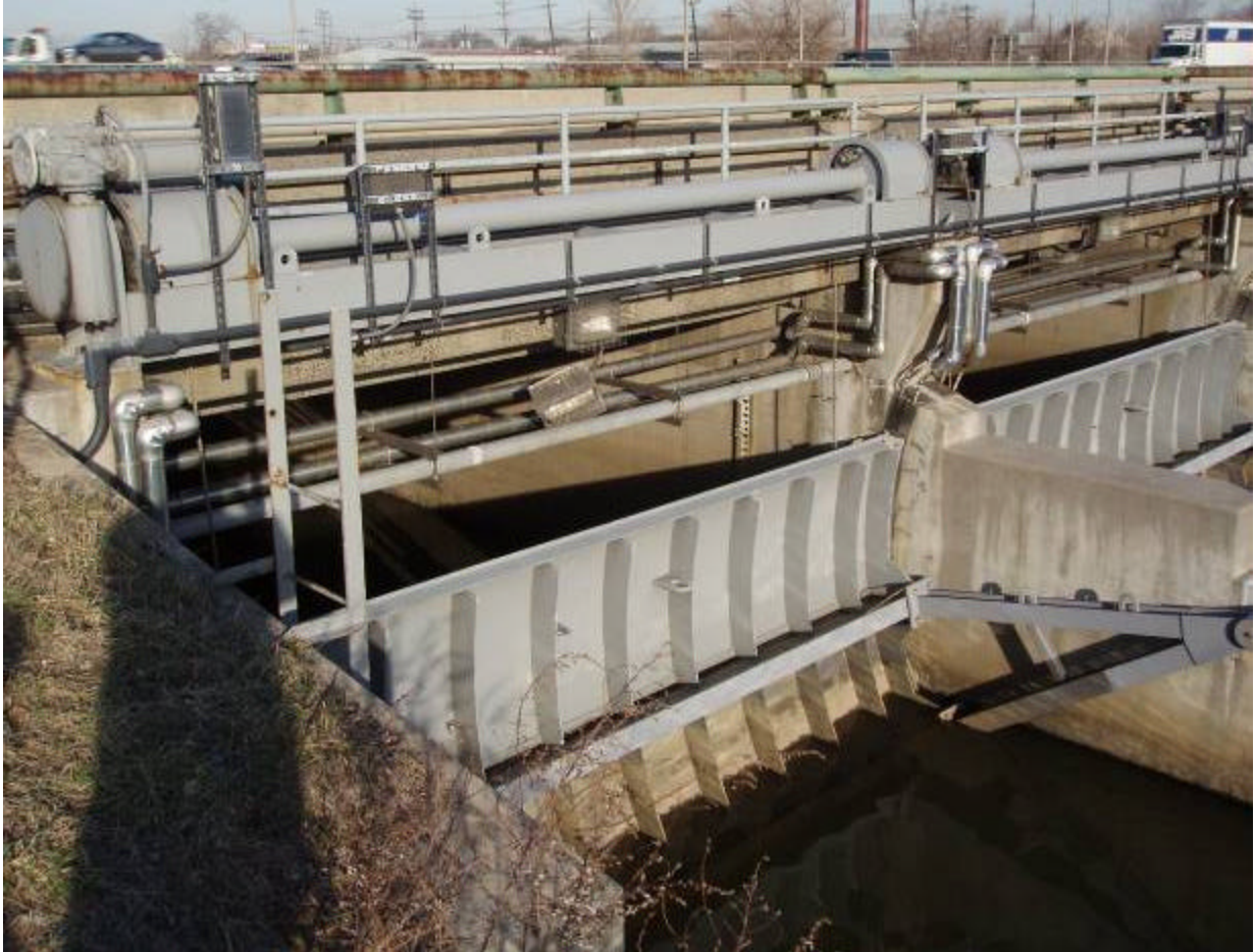
Photo 3 Description: View of bascule tide gate
