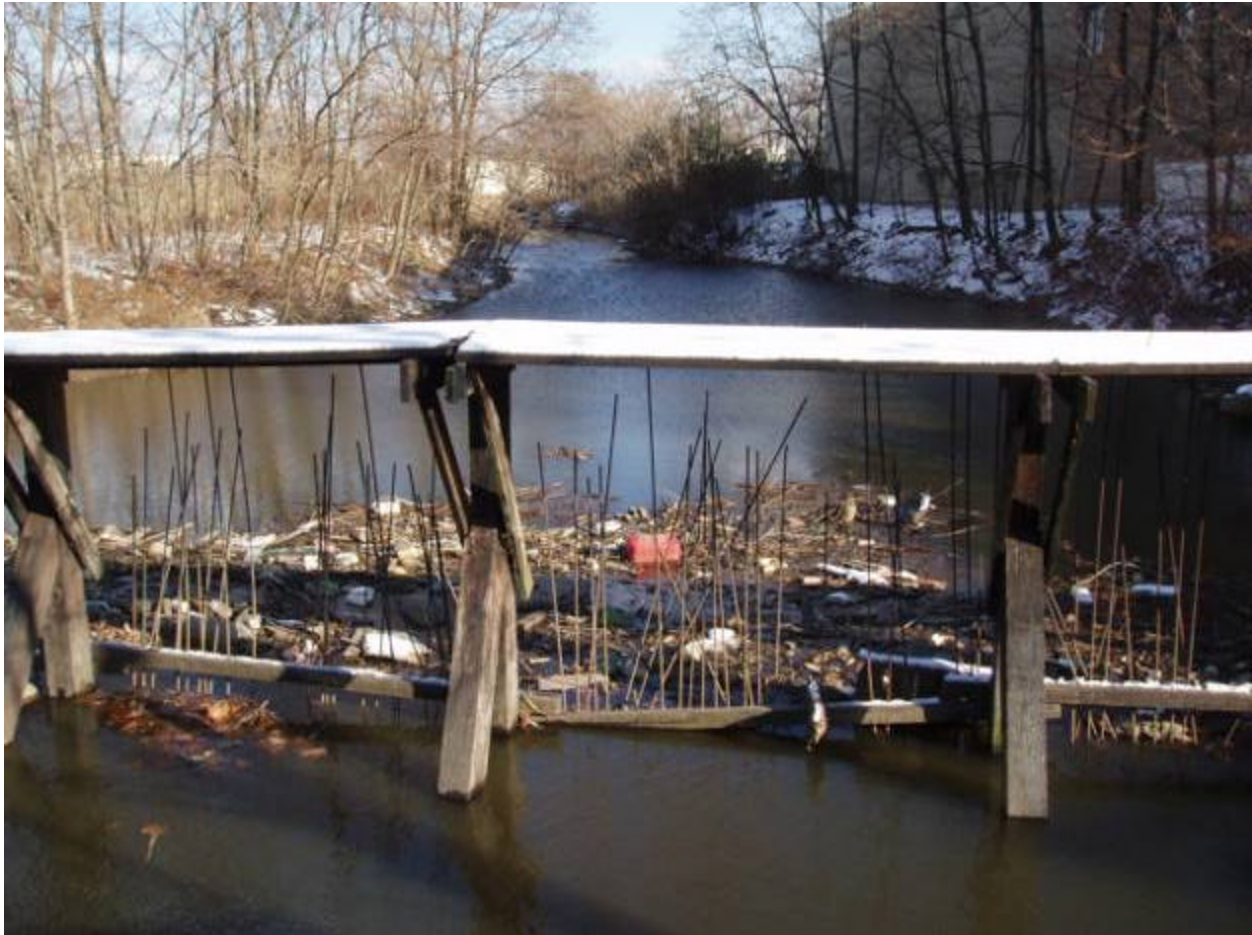
Photo 2 Description: Upstream view from tide gates and view of the trash rack system
