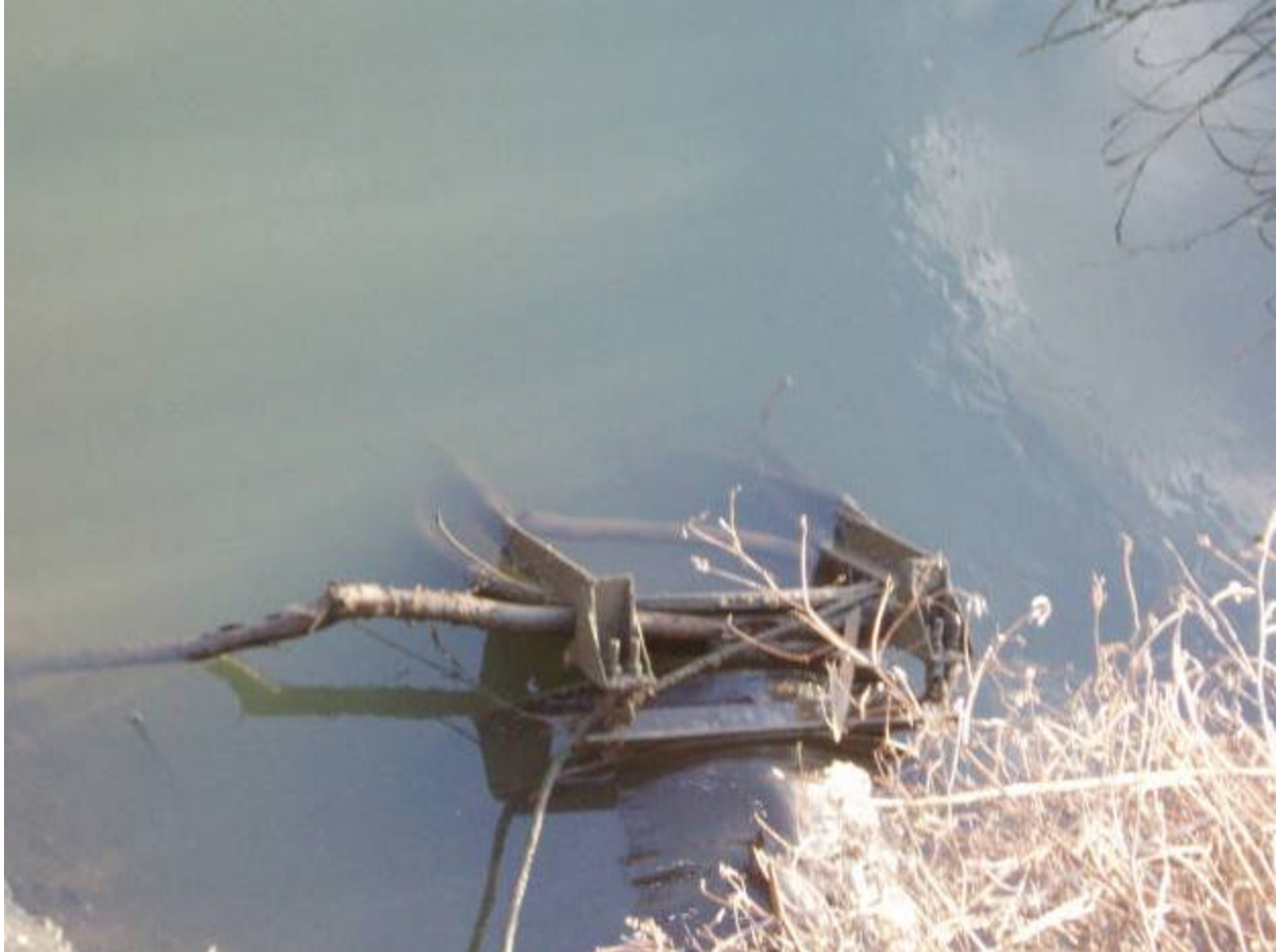
Photo 1 Description: Tide gate shown with debris keeping it from closing properly
