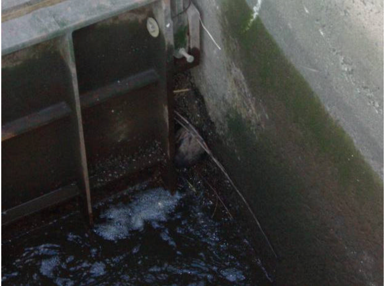
Photo 2 Description: Debris (rock) shown lodged in-between the gate keeping it ajar
