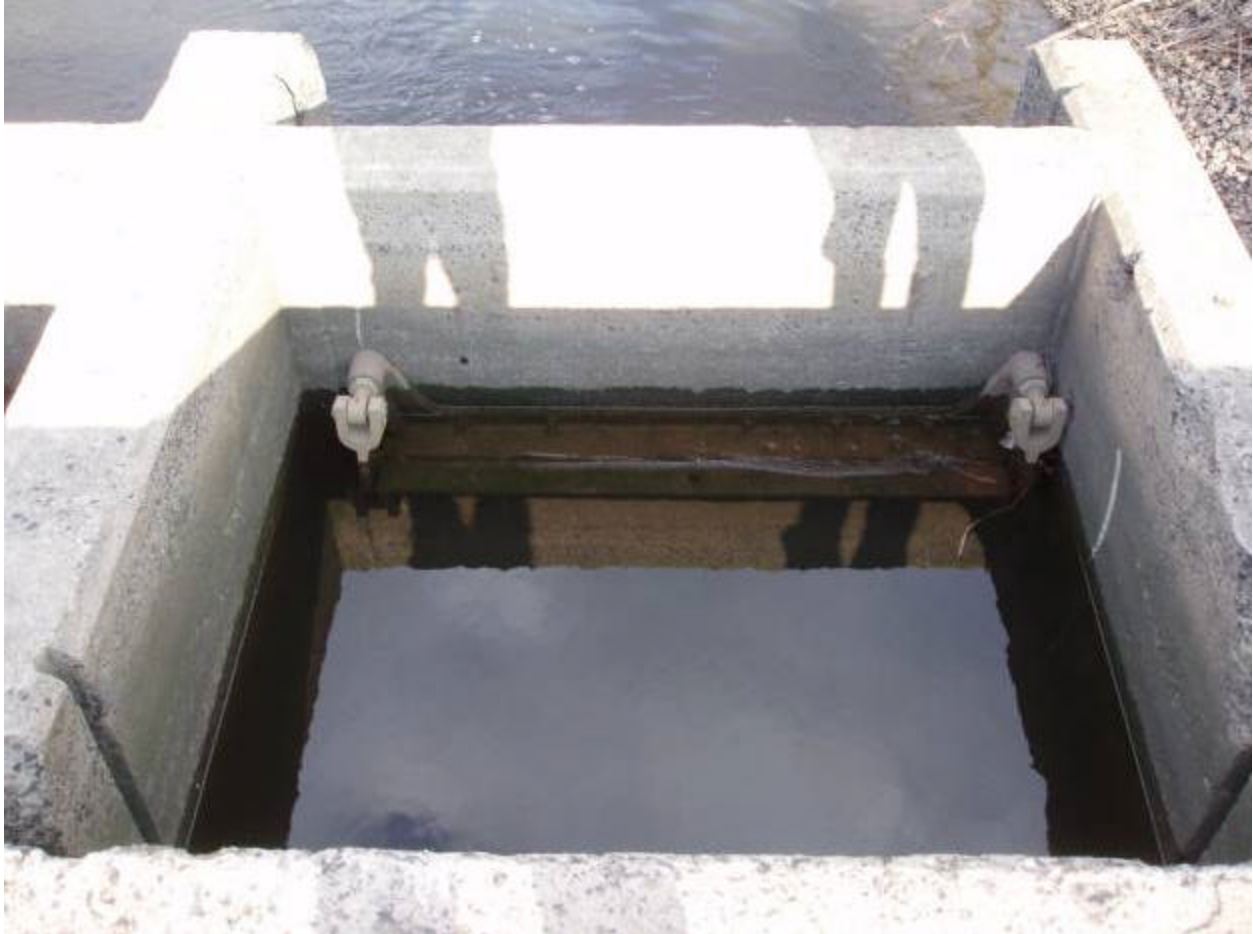
Photo 2 Description: One of two metal flap gates
