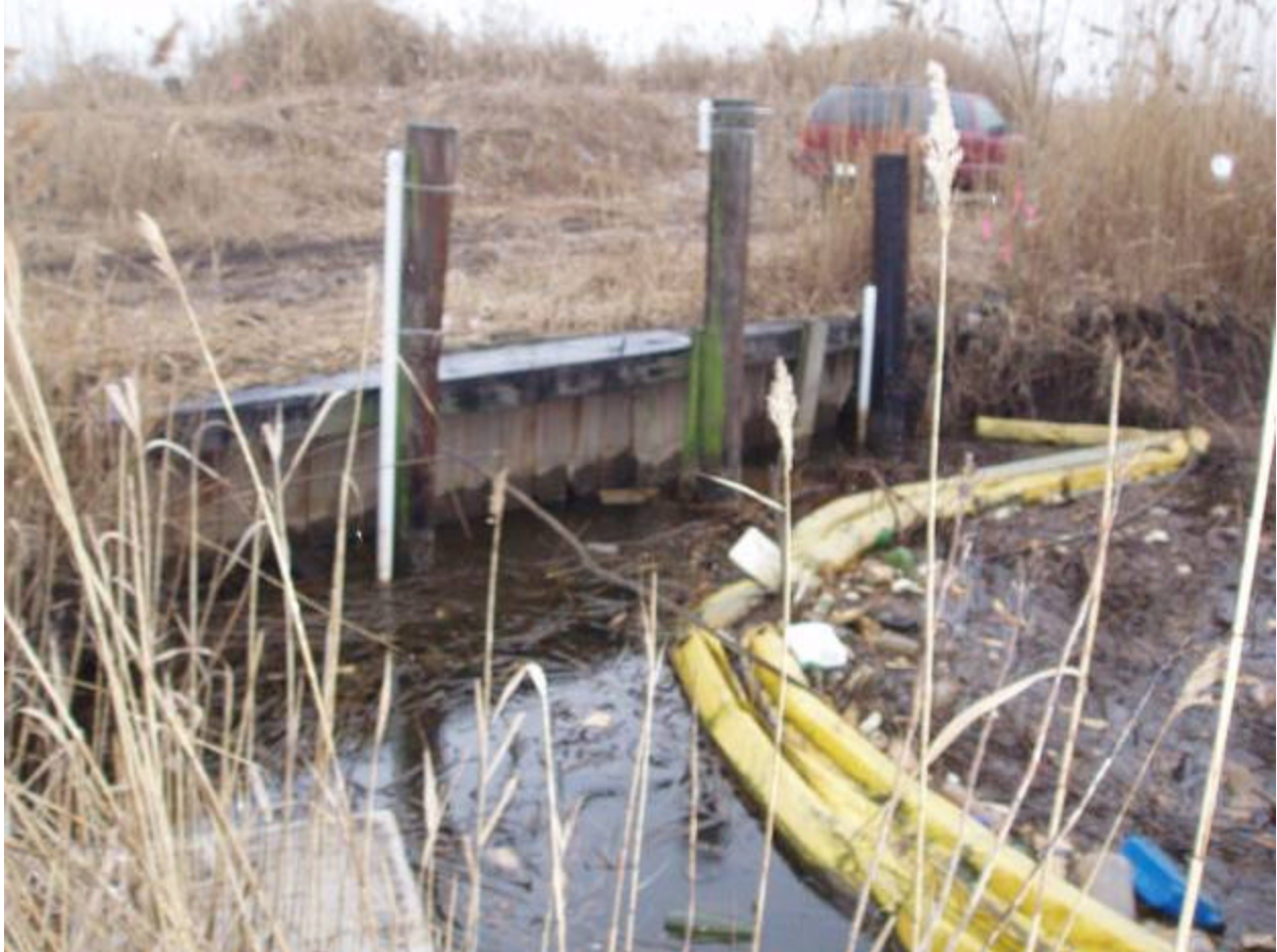
Photo 1 Description: Trash rack system
