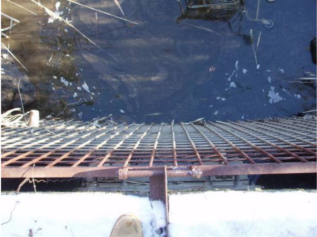
Photo 1 Description: Metal flap gate with a trash rack
