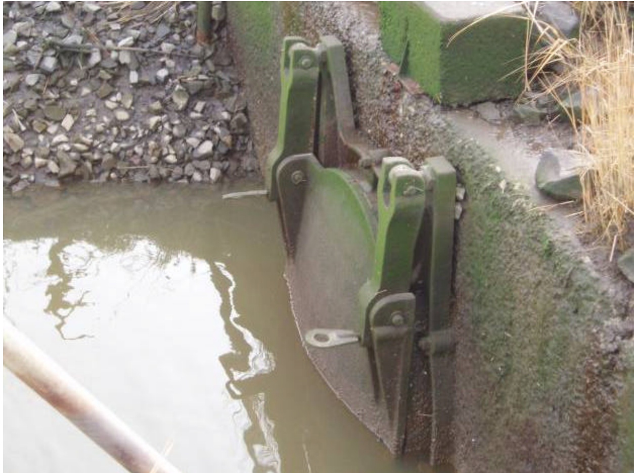
Photo 1 Description: Metal flap gate
