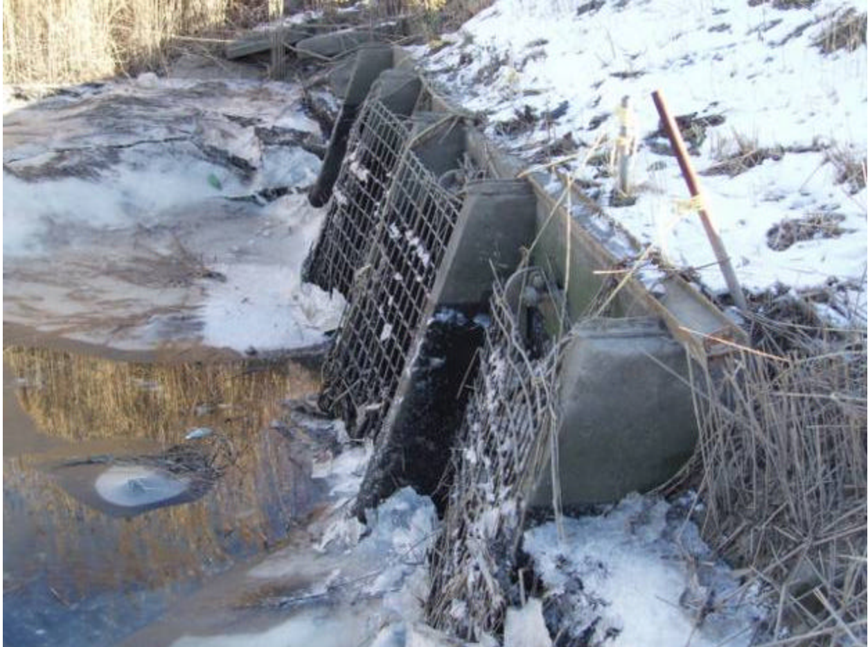
Photo 1 Description: 4 metal flap gates
