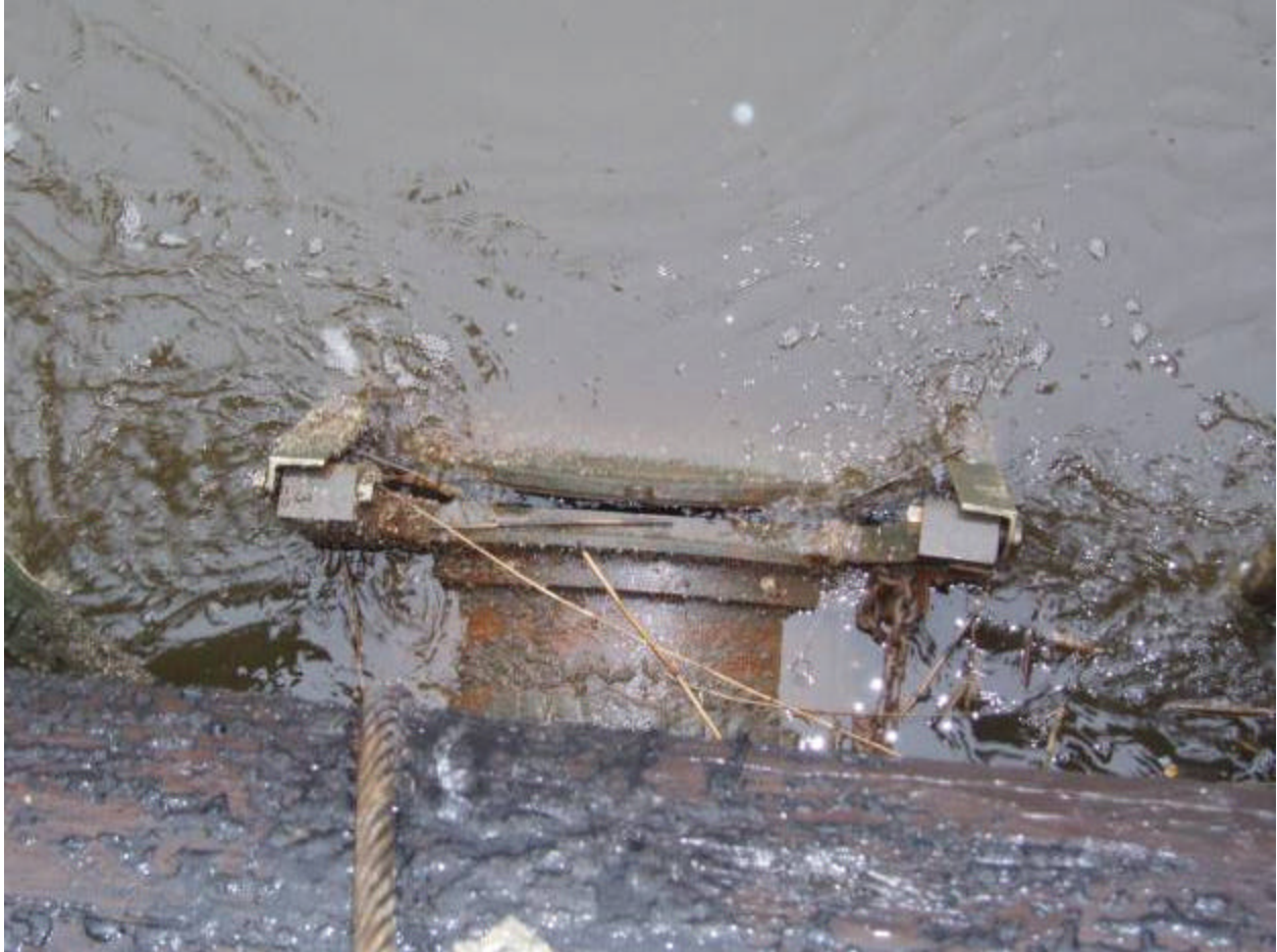
Photo 1 Description: Tide gate shown in the open position
