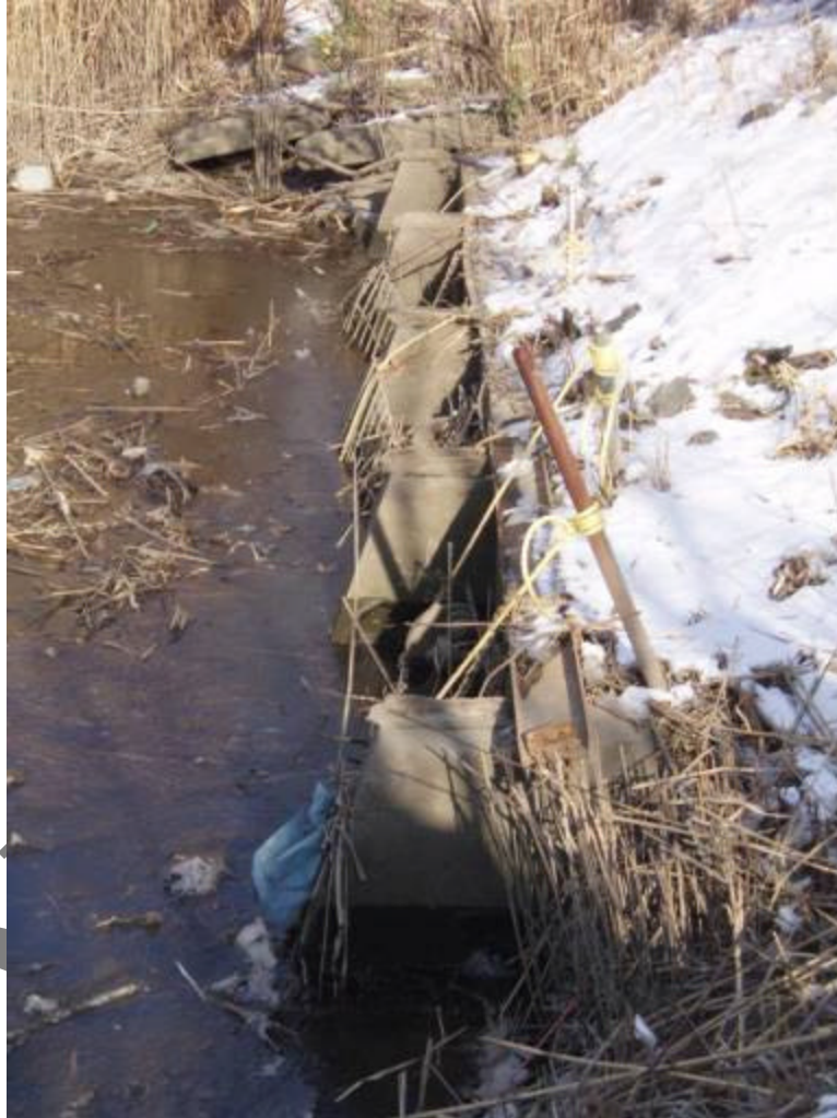
Photo 2 Description: 4 metal flap gates
