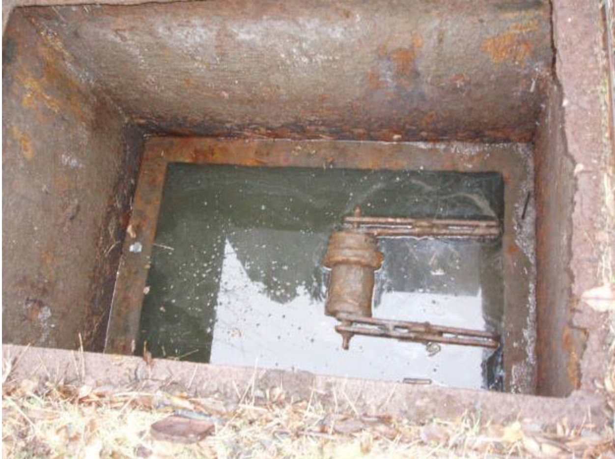
Photo 1 Description: 1 st 30-inch flap gate
