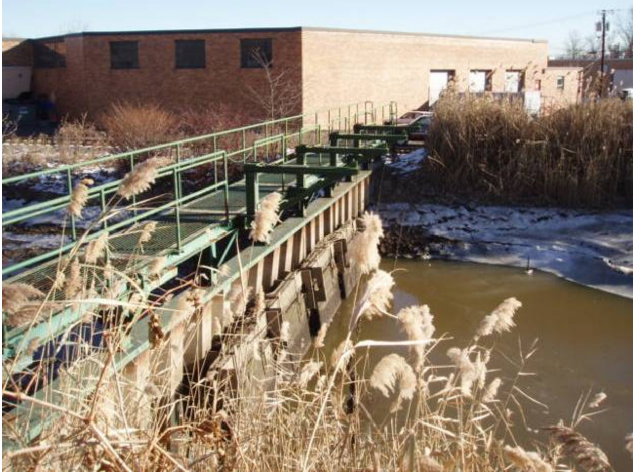
Photo 1 Description: 4 timber tide gates
