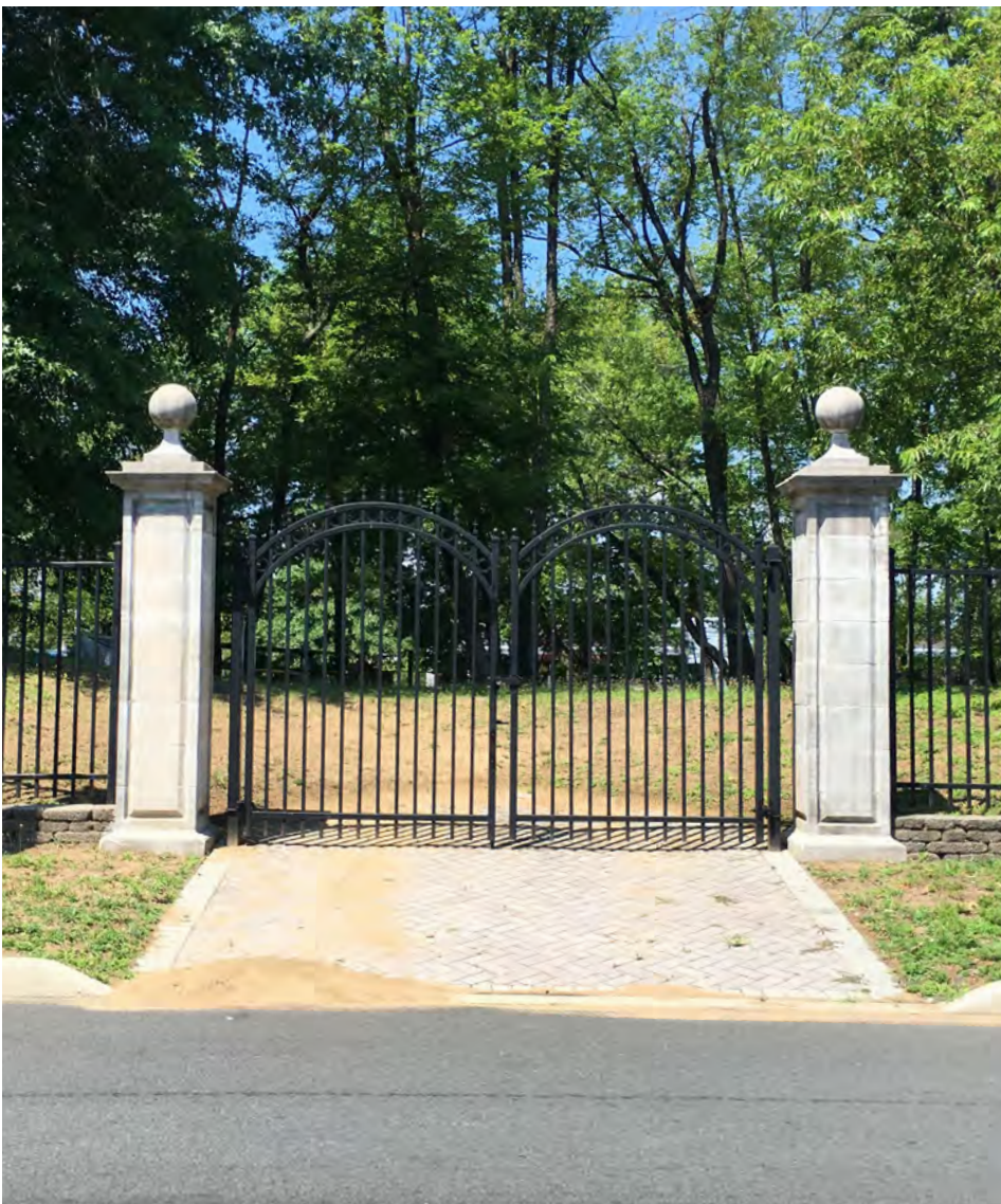
The gated entrance. (Image 3.6.2.2)
