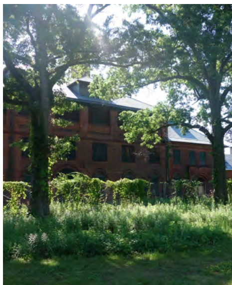
Hackensack Water Works (Images 3.6.4)
