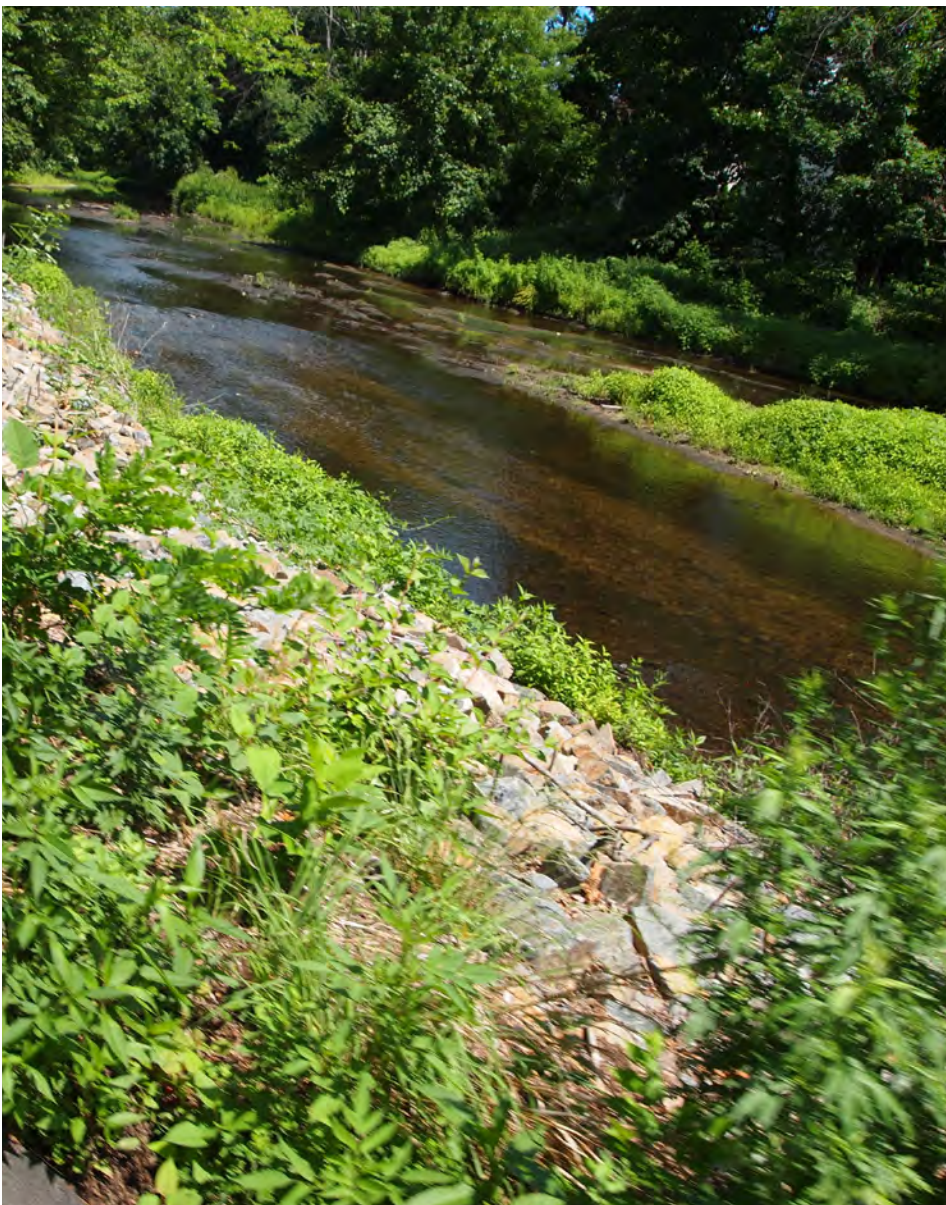
Bank Stabilization (Image 3.1.1.5.2)
