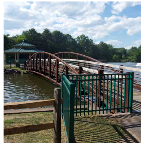
A bridge to the pavilion (Image 3.3.8.3)
