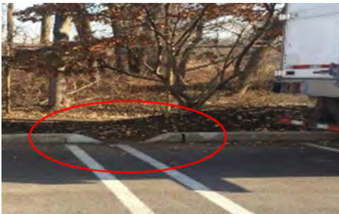
Figure 11. Converting existing curb cuts would help reduce the impact of stormwater on adjacent water bodies (Courtesy of Biohabitats).
