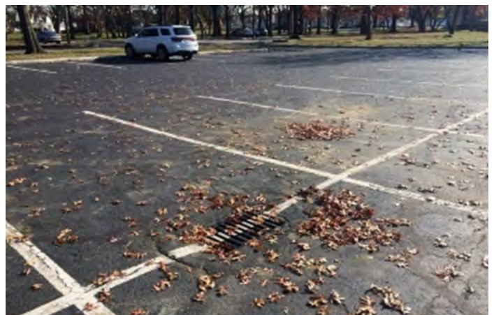
Figure 11. Inlets clog where a small number of inlets serve large drainage areas at Riverside County Park North (Courtesy of Biohabitats).
