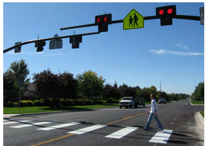
Figure 6. HAWK beacon (Courtesy of BPRC).
