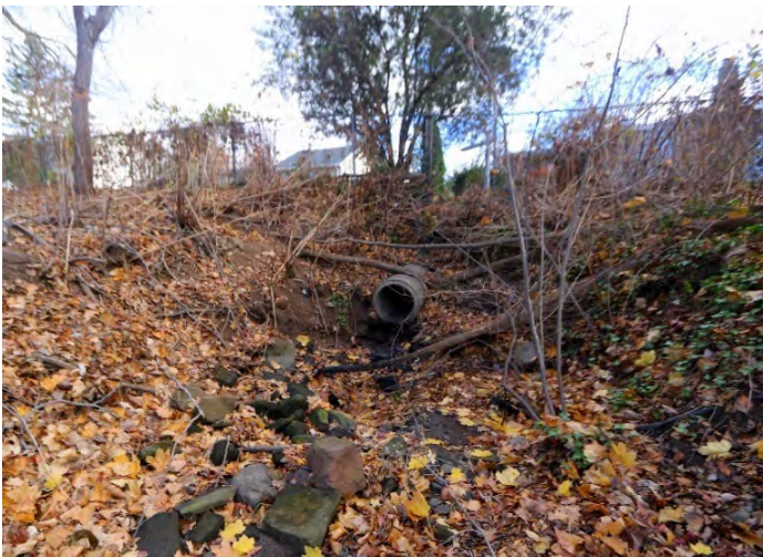
Figure 13. Outfall on steep grade contributes to erosion at Van Saun County Park (Courtesy of Biohabitats).
