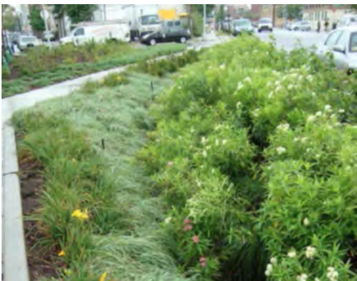
Figure 12. Bioswales help collect, treat and infiltrate stormwater while providing new planted amenities (Courtesy of Biohabitats).
