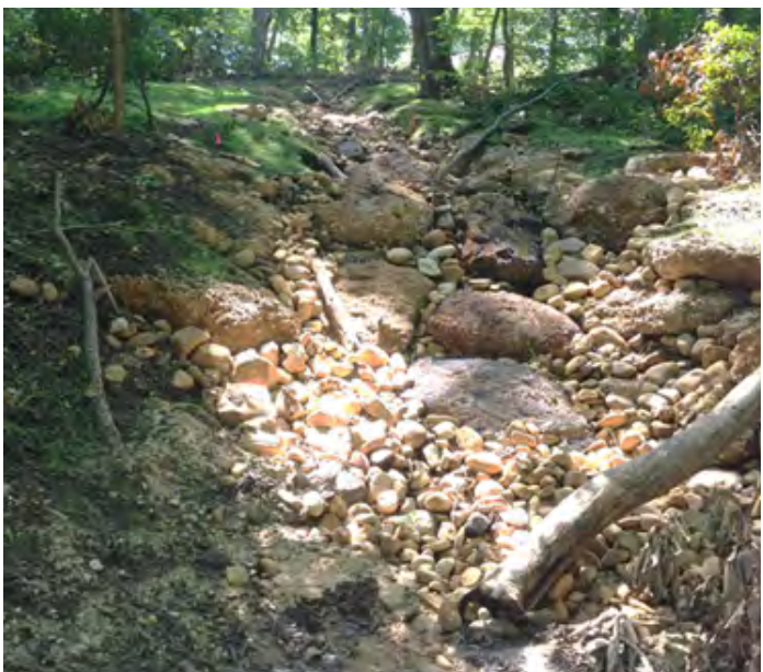
Figures 13 & 14. Existing erosion gullies can be restored using regenerative stormwater conveyance techniques to slow and retain stormwater (Courtesy of Biohabitats).
