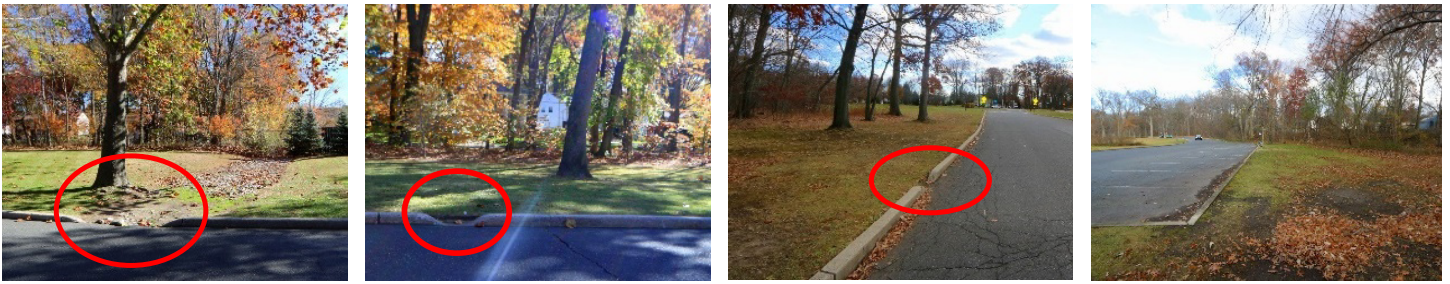
Figure 6A-D. Curb cut and concentrated sheet flows contribute to isolated ponding and sedimentation in Van Saun County Park (Courtesy of Biohabitats).
