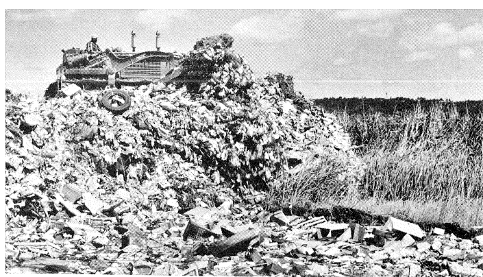
REFUSE, compacted by hydraulic fill, lies beneath Overpeck Bergen County Golf Course. (Before and after photos above.) The golf course was the first major recreation facility developed on the marshy Overpeck County Park site.
