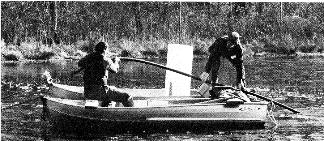
AERATION equipment is installed at the Bergen County Wildlife Center to keep the pond clear.
