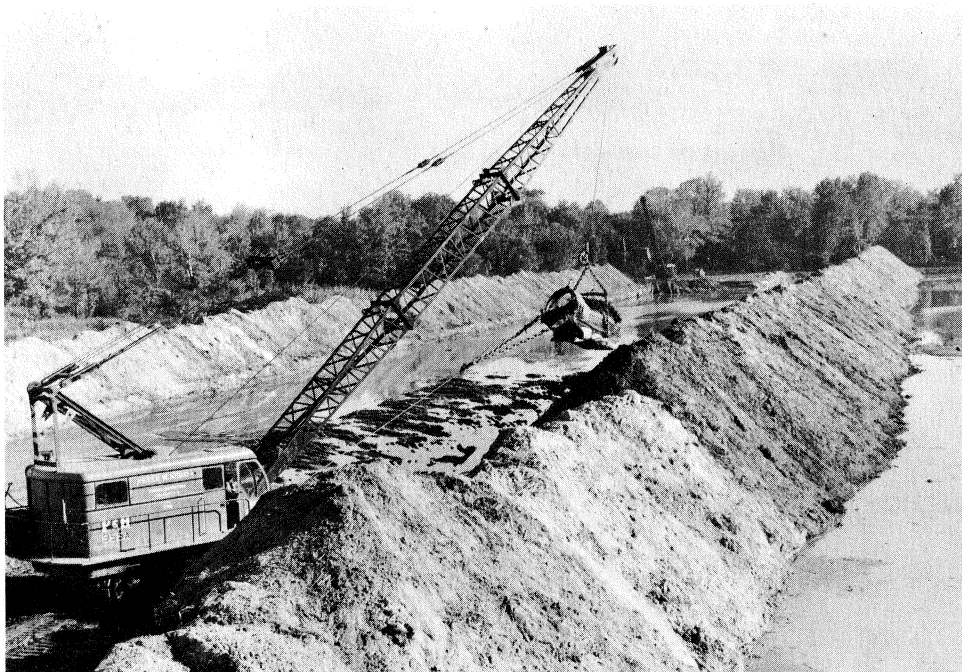
Virgin meadow topsoil is stockpiled in ridges 15 feet high for the golf course to be built in Overpeck County Park.
