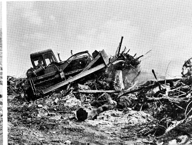
The Commission's bulldozers start to clean up the area. A disposal method known as Sanitary Land Fill will be carried on.
