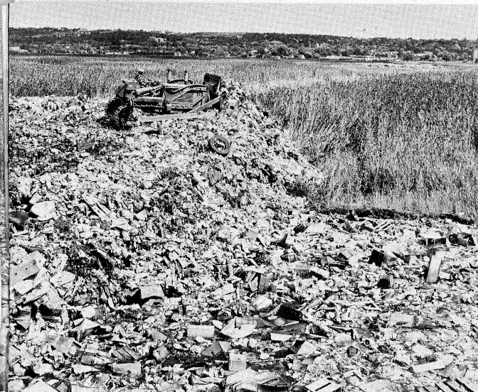
Piles of refuse are leveled and made more available for burying. The above pictures were taken in the Ridgefield Park area.
